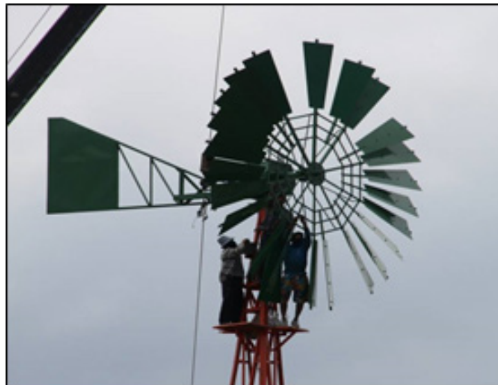
Figure 8. Installation of the multi-blade wind turbine
